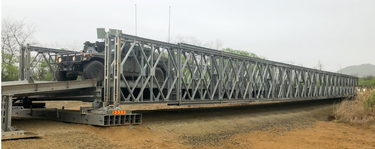
Figure 3. A humvee from 3/1 ABCT crosses a 40-meter LSB over a dry gap constructed by members of 814 th MRBC. (U.S. Army photo by LTC Robert Dion)
