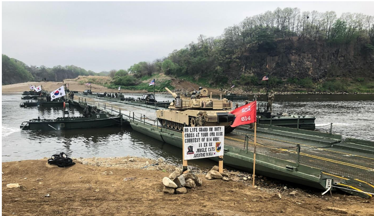
Figure 2. An M1A2 tank from 3/1 ABCT crosses a hybrid IRB/SRB bridge constructed by members of 814 th MRBC and 6 th Engineer Brigade (RoKA) during a wet-gap crossing exercise. (U.S. Army photo by LTC Robert Dion)
