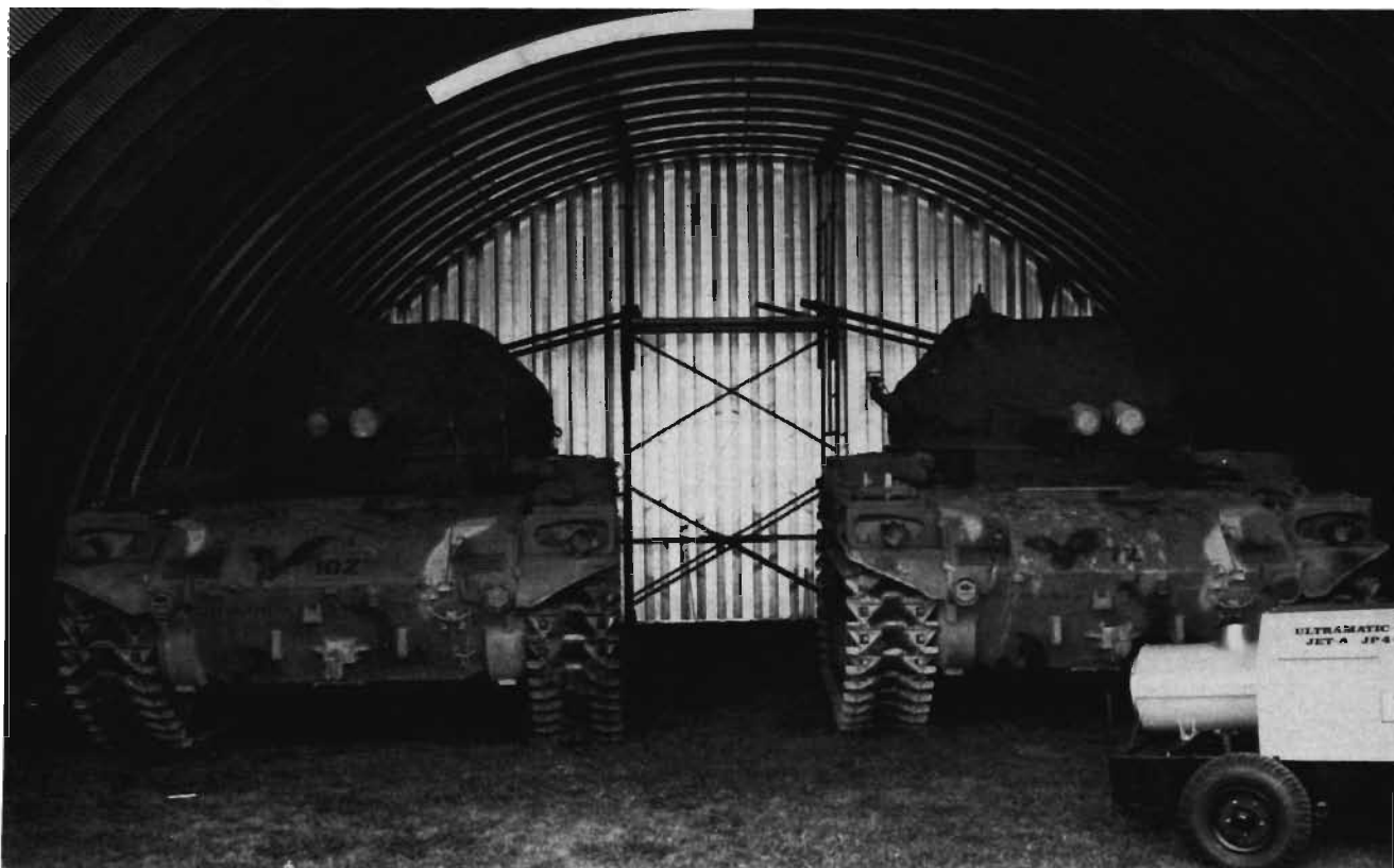
"Quick-Fix" building interior showing a pair of "Duster" twin 40-mm antiaircraft vehicles. The 50-by-35-by-17-foot building was erected by six men in eight hours, using only common tools. Erected at Fort
