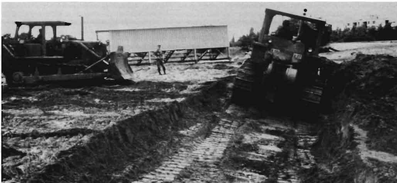
Two bulldozers working together to cut a tank bump obstacle. One cuts the V-shaped ditch while the other builds the berm.
