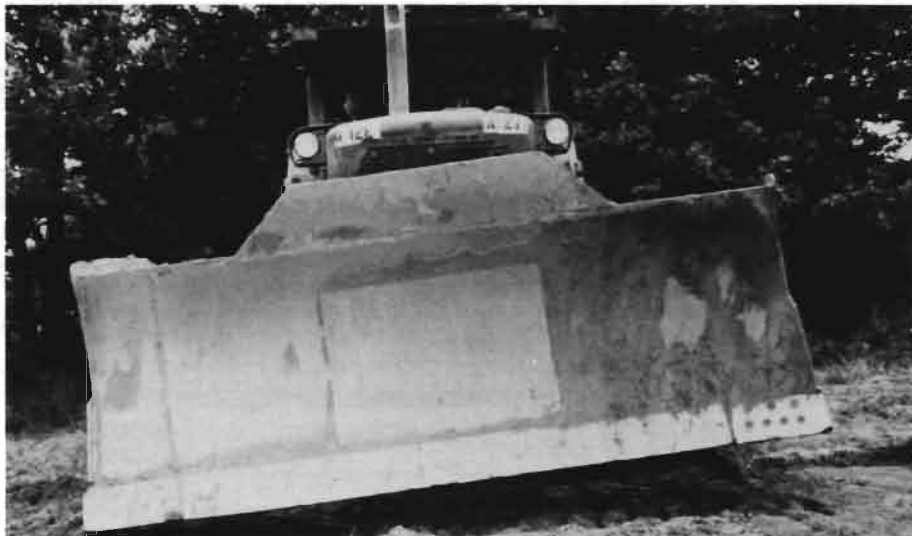
A bulldozer must be used to cut the ditch because its blade can be angled to create the V-shape needed.
