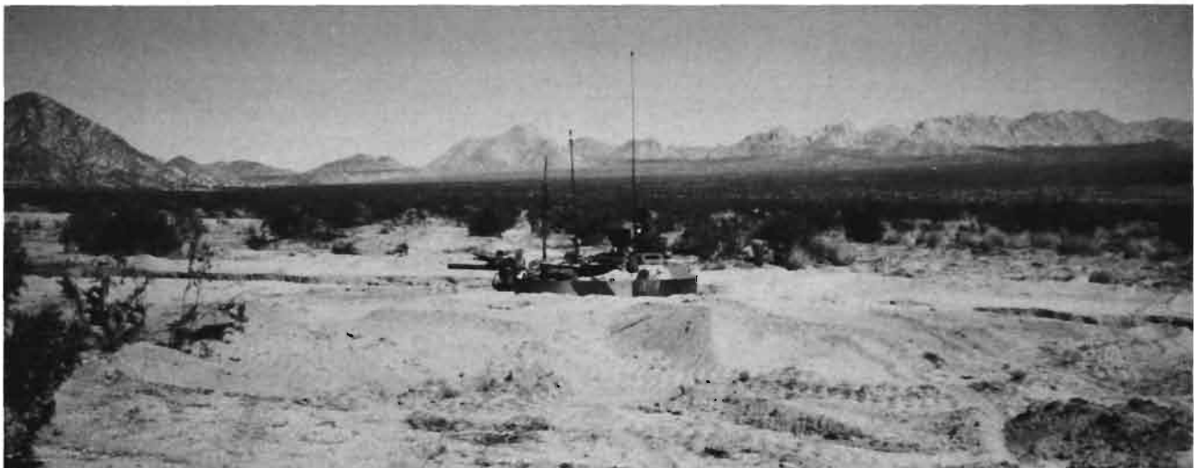
A typical OPFOR fighting position for a BMP is constructed in two tiers, allowing the vehicle to hide in turret defilade and fight from hull defilade.
