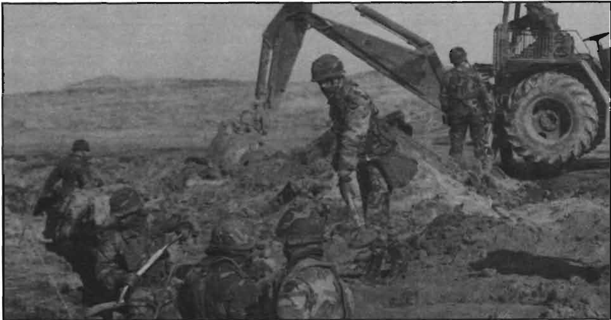
Excavators can loosen soil, even if there's not enough time to finish the job by machine.
