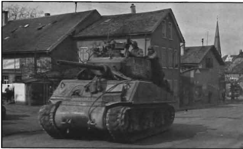
SHERMAN M4A3E2 "JUMBO" WAS FIELD-CONVERTED TO HIGH-VELOCITY 76-MM GUN, CARRIED MORE ARMOR, AND WAS EQUIPPED WITH TRACK EXTENDERS.
