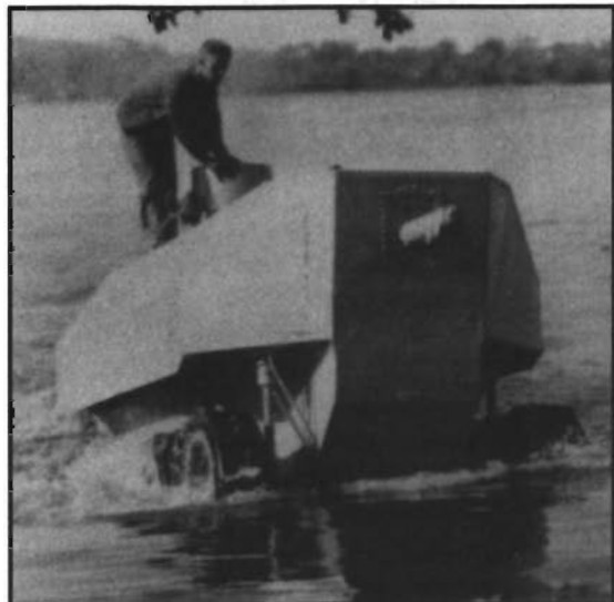
In the photo at left, Marines of 8th Company, 5th Regiment, test the Christie Marine tank's assault capabilities in late February 1924, at Chiriqui Lagoon, Culebra, Puerto Rico.
