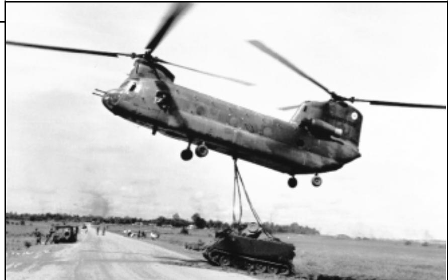
*"Supporting armor requires BIG birds, not utility choppers.... One Chinook...can lift a basic load for a tank, AGS, or Bradley platoon, plus a couple of fuel bladders, MREs and the mail. What is needed is an air troop with CH-47s, and this opens up a whole new box of capabilities."*
