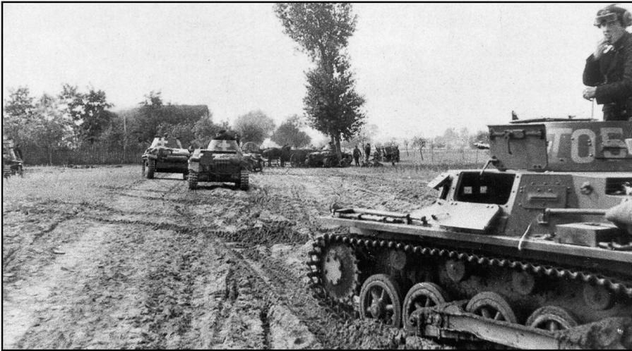
German armor employed in Norway was similar to these tanks photographed during the earlier invasion of Poland. Here, a Pzkw I, foreground, acts as a command tank for the Pzkw IIs in the background. Both light tanks, they were armed with machine guns and in the case of the Pzkw II, a 20mm automatic cannon.
