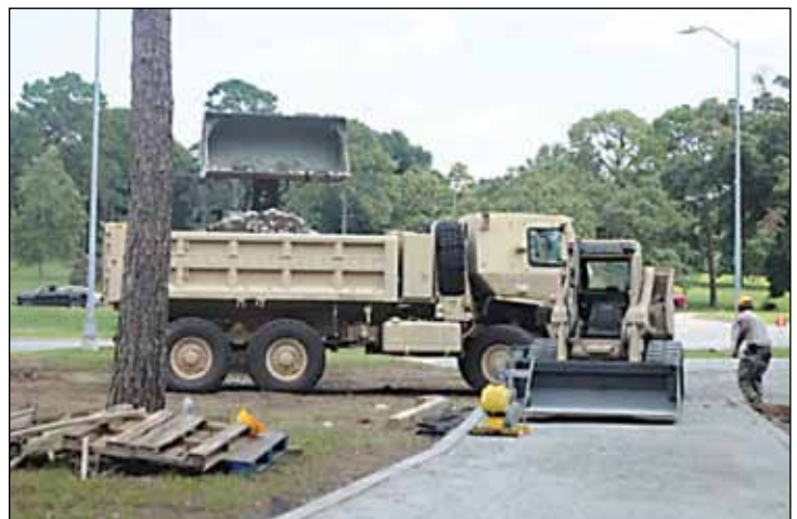
Soldiers from the 7 th Battalion, 18 th Engineer Company work on a trail and parking lot for Pattons’ Park. The park will feature a continuation of artifacts displayed in the Armor and Cavalry Gallery in the National Infantry Museum.
