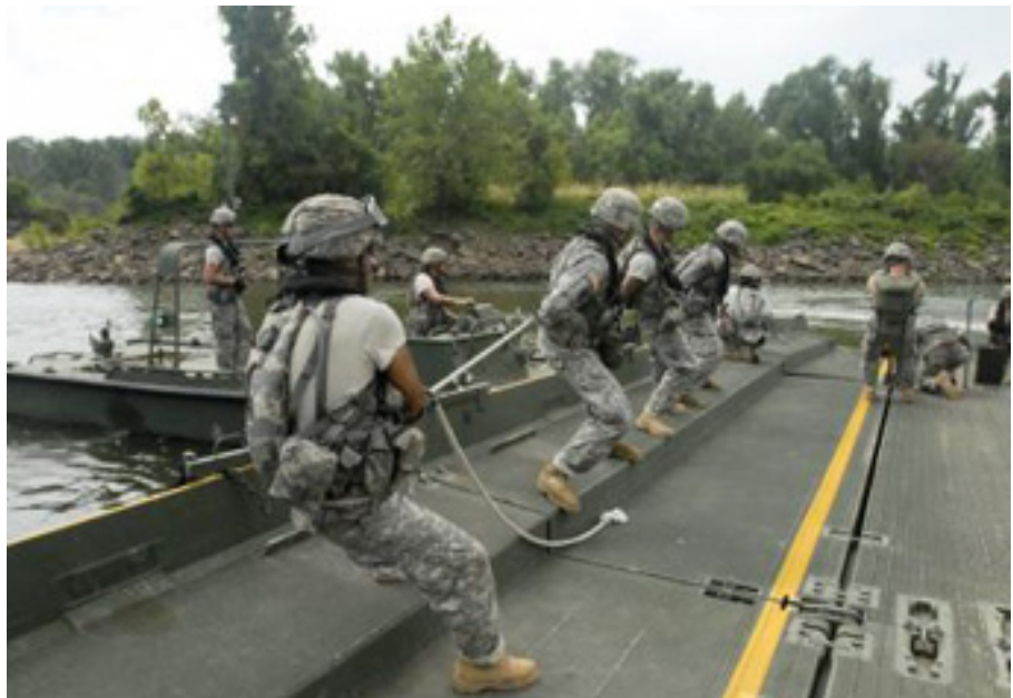
Figure 3. U.S. Army Reserve Soldiers of 652 nd Engineer Company, located in Hammond, WI, remove tension in bridge bays before disconnecting them on the Arkansas River as part of a training event at River Assault 2011 at Fort Chaffee, AR, July 26, 2011. The exercise culminated in the construction of a floating improved ribbon bridge across the Arkansas River. Resources and partnerships can be trained after proper CoA development. (U.S. Army photo by SPC Brittney Bradley, 343 rd Mobile Public Affairs Detachment, source: http://www.dvidshub.net/image/435931/river-assault-bridge-crossing#ixzz2mzl8jYm7 )
