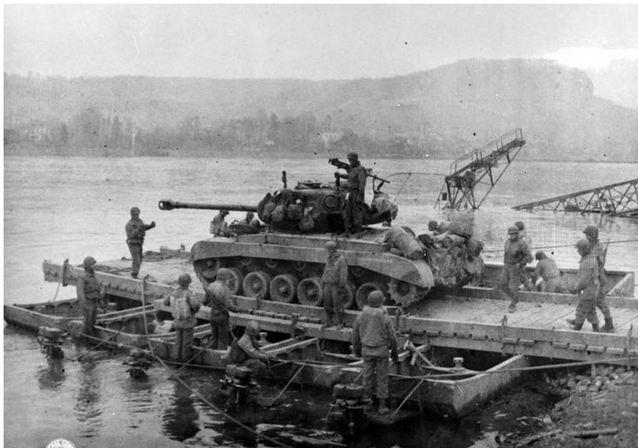
**Figure 4. An M26 Pershing T26E3 from Company A, 14<sup>th</sup> Tank Battalion, is transported aboard a pontoon ferry across the Rhine at Remagen March 12, 1945. The ferry was built by 1<sup>st</sup> Engineer Heavy Pontoon Battalion. (U.S. Army Signal Corps photo)**
