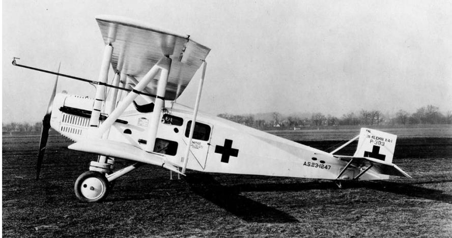
**Figure 3. An example of an interwar “ambulance airplane.” This was the only type of airplane capable of operating from unimproved airfields to evacuate casualties from near the front, but it was vulnerable to navigational errors, bad weather and enemy air defenses. (Reeve photograph collection, Otis Historical Archives, National Museum of Health and Medicine)**
