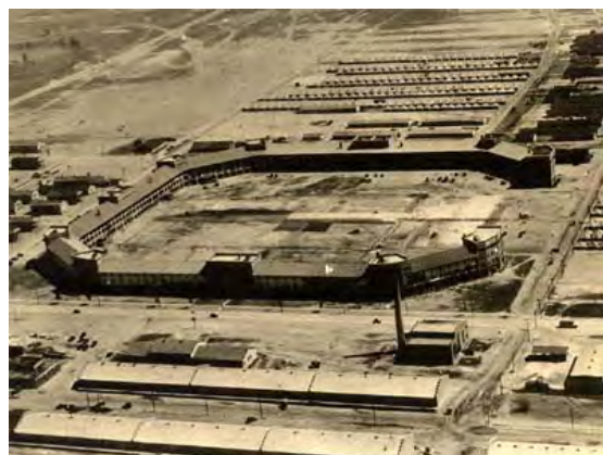
The Cuartels under construction (circa 1925)
