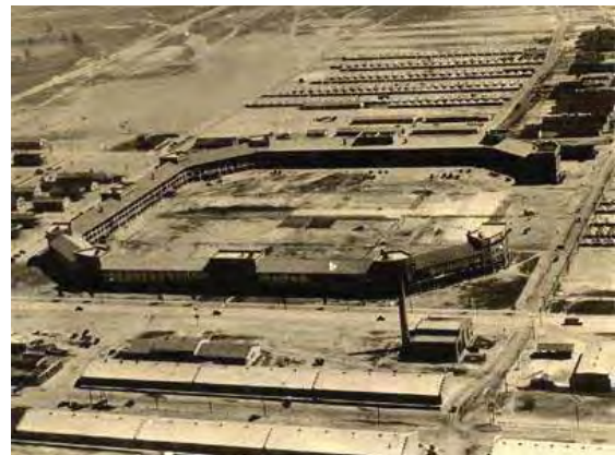
The Cuartels under construction (circa 1925)
