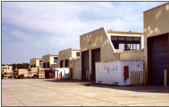
Existing Maintenance Bays
